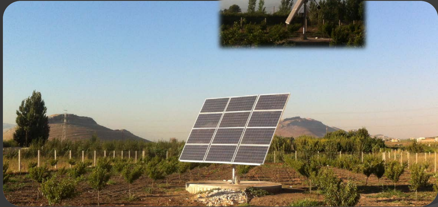
Residential solar system with PV tracker
