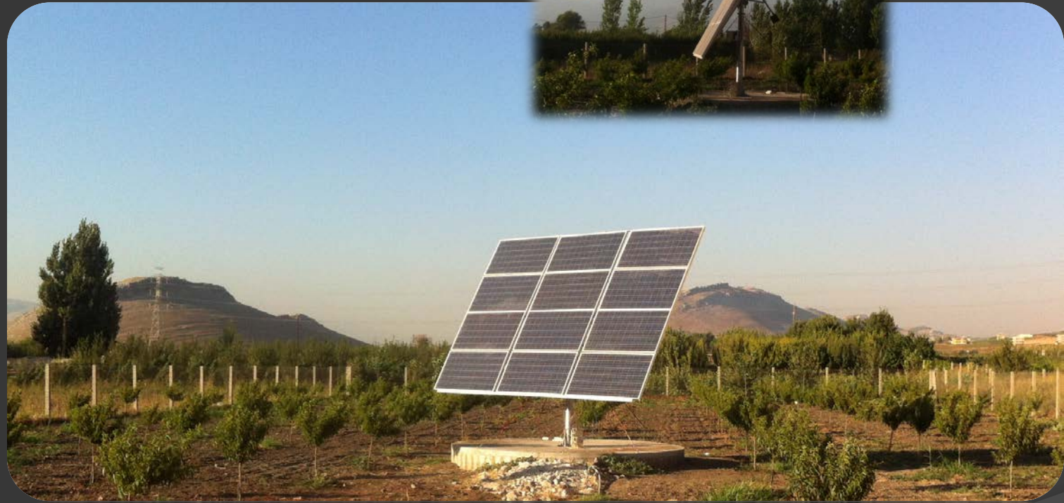
Residential solar system with PV tracker
